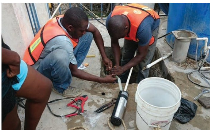
Haiti ICT Lucson Celestin works to install a new submersible pump at Eglise Episcopale Saint Esprit de Anotte in Cavallion, Haiti, after Hurricane Matthew.
